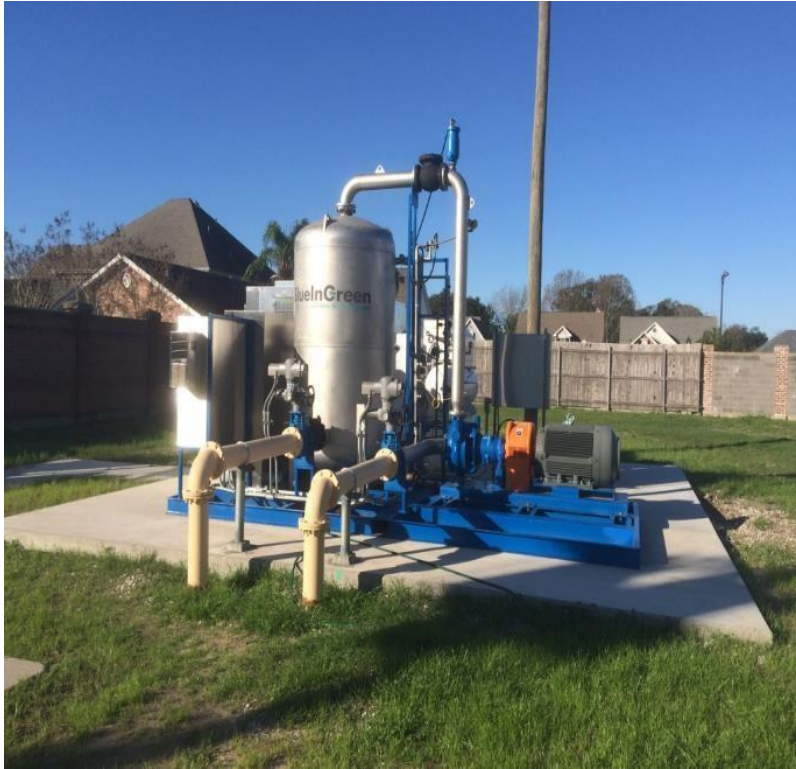
Lift Station : G6-9 Helios SDOX-CS 600 SDOX-CS 1000 2,000-lb/d 8,000-lb/d 800-gpm
