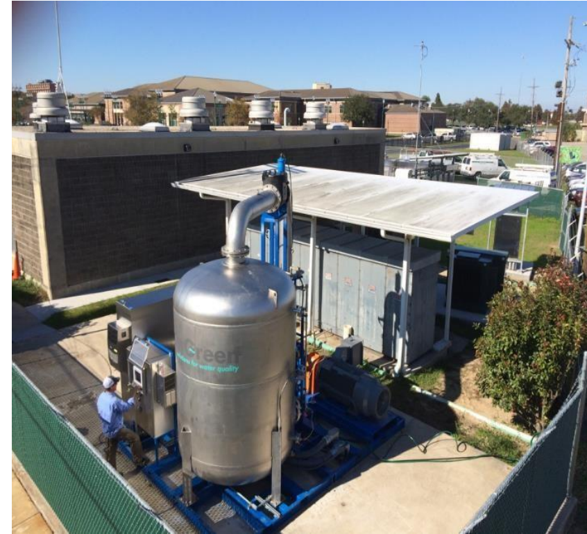
Lift Station : G6-9 Helios SDOX-CS 600 SDOX-CS 1000 2,000-lb/d 8,000-lb/d 800-gpm
